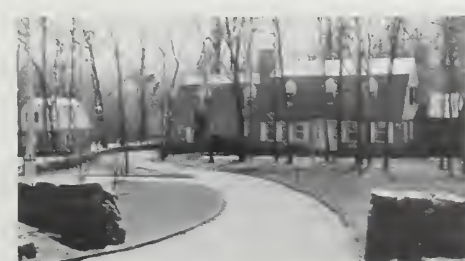
Main residence and guest house
